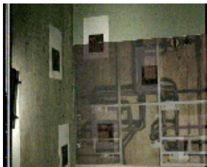
Figure 8: Same room after completion, showing the real dry wall with a semi-transparent augmentation of the piping in the wall.
